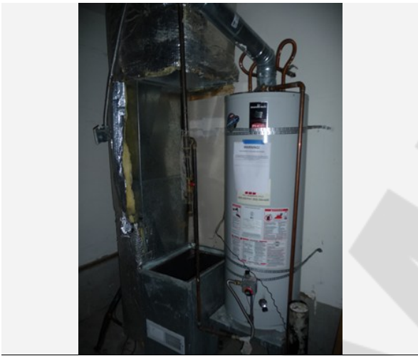
Area: Systems Repair For: Heating - Forced Air
