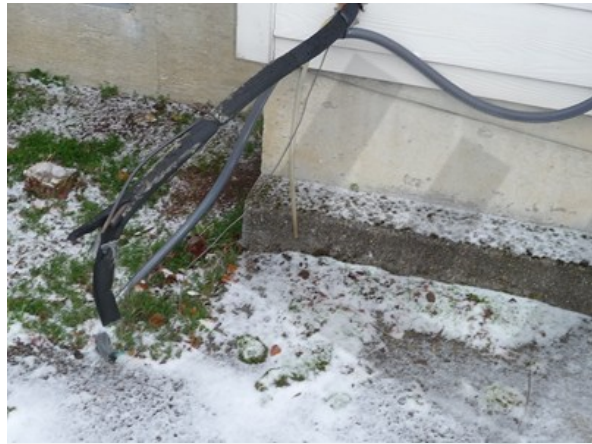
Area: Systems Repair For: Cooling - Central A/C
