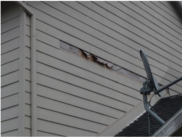
Area: Main Structure Repair For: Exterior Walls - Wood
