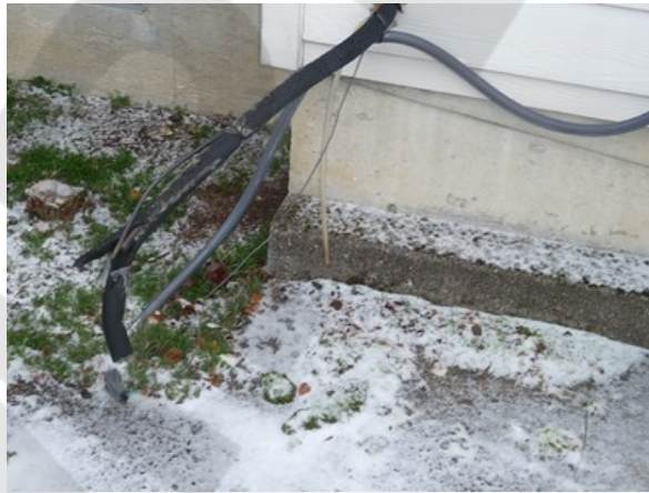
Area: Systems Repair For: Cooling - Central A/C
