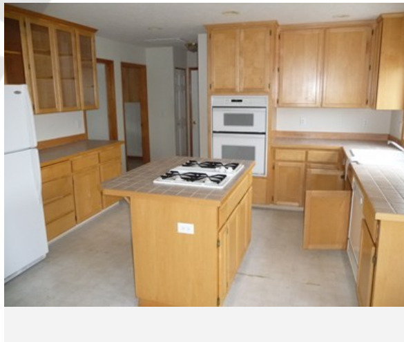
Area: Kitchen Repair For: Flooring & Steps - Vinyl
